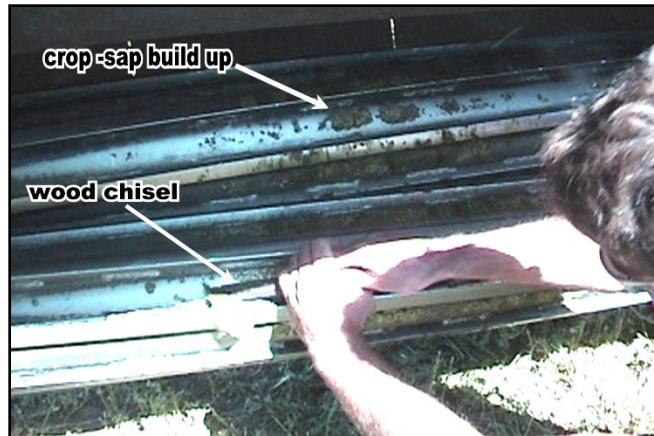
FIGURE 39 SCRAPPING BUILD UP FROM ROLLER
