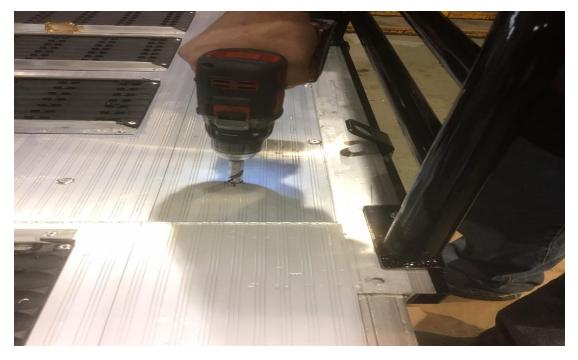
3. Place the front support leg into position and install the 2 -  $5\frac{1}{4}$  bolts with washers and nyloc nuts (do not tighten).
