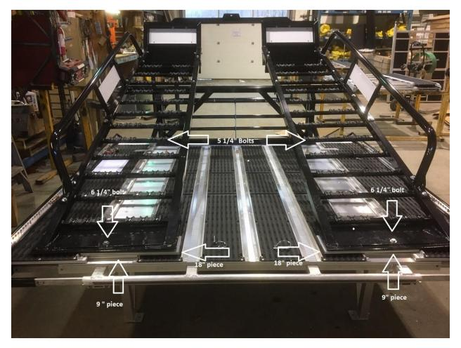
4. Install 2 – 6  $\frac{1}{4}$  bolts with 2 flat washers and nylocs. Thru the deck pad as well as the 18" and 9" spacers and thru the deck.
