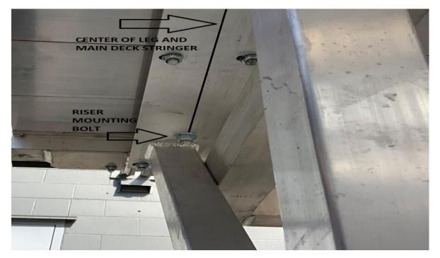
2. Drill 9/16" hole (start with ¼" pilot hole as you are drilling thru 4 layers). Repeat on other side.
