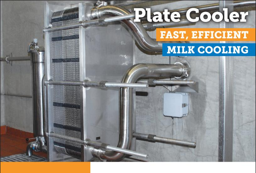
BouMatic Plate Coolers are unrivaled for fast, efficient milk cooling and will use your well water or chilled water for the most effective milk cooling.
