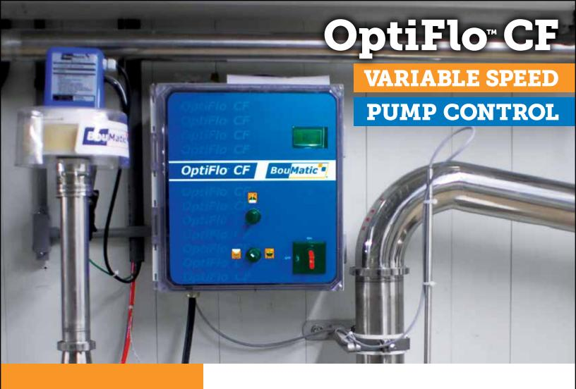
The only true variable speed milk pump control giving you the ultimate in cooling system efficiency. Optimizing the milk flow rate through the plate cooler for the best cooling system performance.
