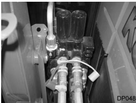
Figure 12 Remote Control Valve Hoses
