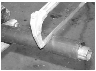
Figure 3. Cut Shield
