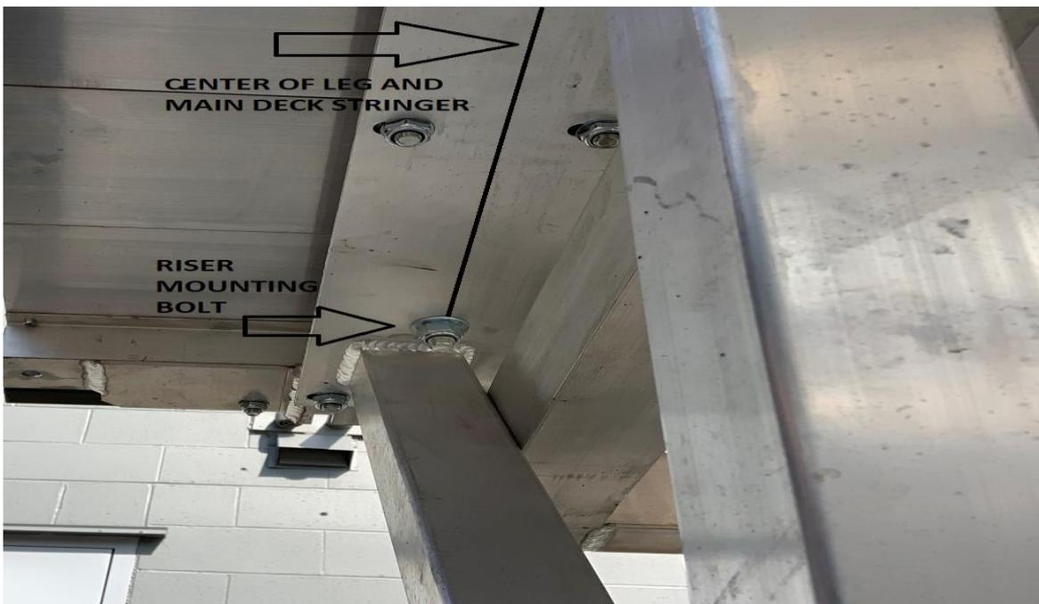
2. Drill  $9/16''$  hole (start with  $1/4''$  pilot hole as you are drilling thru 4 layers). Repeat on other side.
