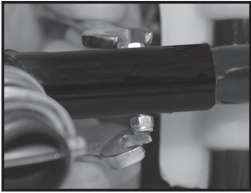
Figure 4 Tighten nut to bolt
