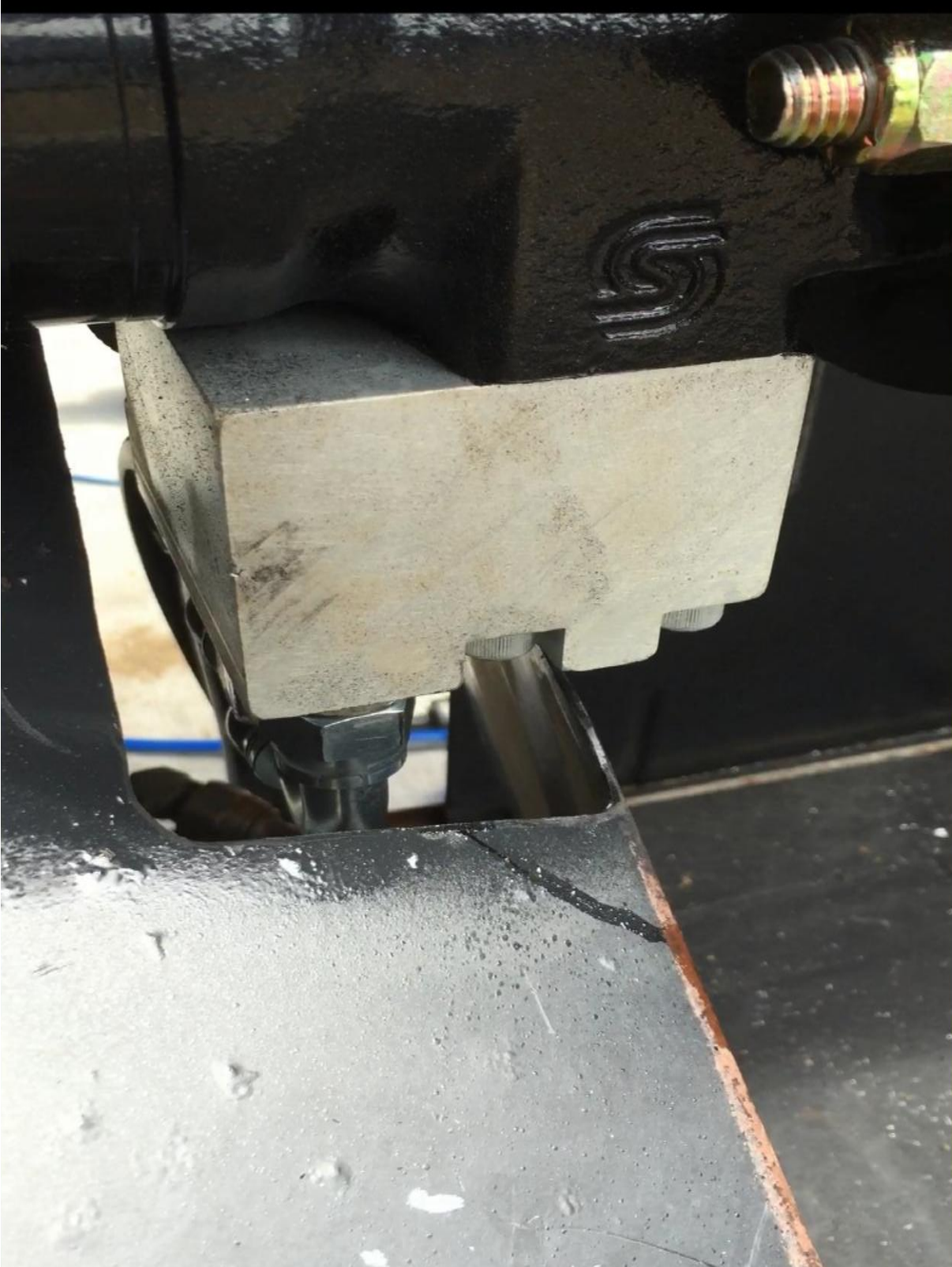
Notch tin in side of header for motor to fit in.
