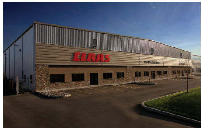
The CLAAS Parts Logistics Center in Regina Saskatchewan, stocks more than 14,000 part numbers in a warehouse area of over 33,000 sq ft.
