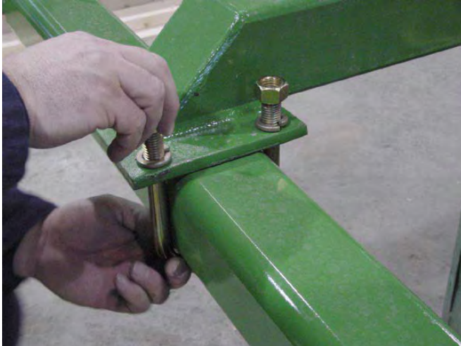
22. Secure Cross Braces.
