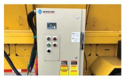
MOTOR STARTER PANEL. The motor starter panel provides a variable frequency drive (VFD) panel.
