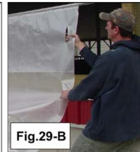
**31.** The curtain can now be raised until the top limit is reached. This is achieved when 3" of the curtain overlaps the header using an electric drive. The limit switch will be set.
